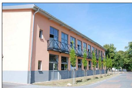
The workshop consists of a long, two-storey production hall and a smaller building containing the cafeteria on the ground level and sanitary facilities on the upper floor. Connecting the two is a glass and steel entrance hall/lobby with a lightweight staircase.
